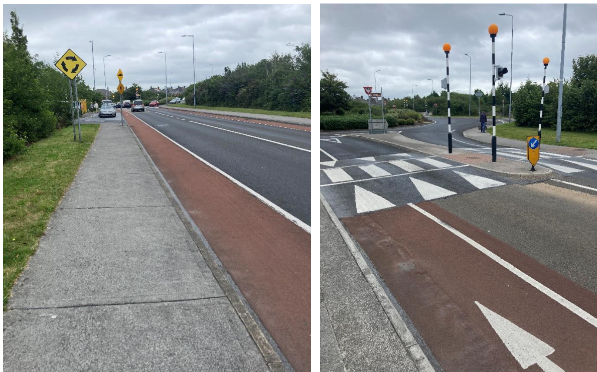
Figure 2-5 Western Distributor Road
