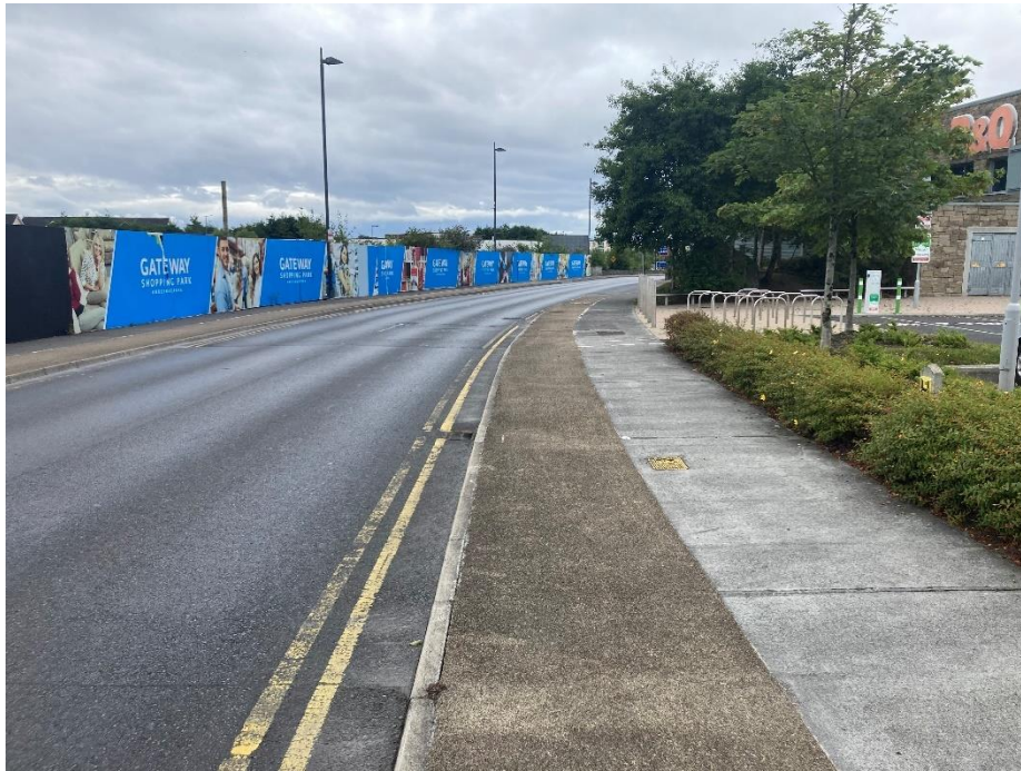
Figure 2-10 Gateway Retail Park internal link road
